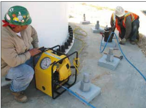
◀ *The ZUTP-1500 pump is rugged, lightweight, compact for tight openings, and delivers hassle-free operation of bolt tensioning in remote locations with up to two times the speed of competitive pumps.*
