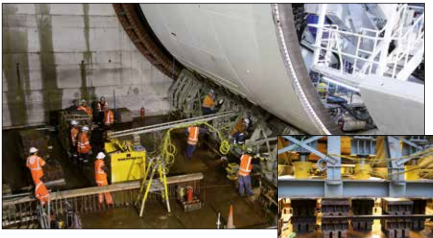
▼ 3600 ton Tunnel Boring Machine lowered and tilted into its starting position with the EVO-Series Synchronous Lifting System.
